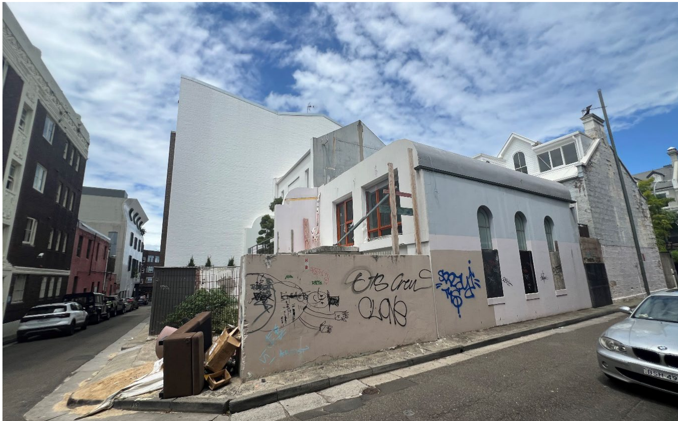
residential terrace (under construction) on opposite side of Kellett Way
